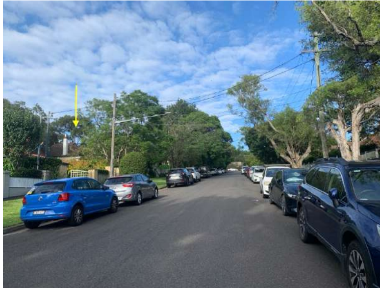
Figure 36: View towards the heritage item, marked by the arrow, on approach up Middle Harbour Road from the north east. The side of the roof and chimney of the heritage listed dwelling are visible. The item is not prominent on approach in this direction.
