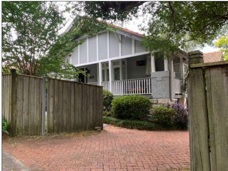
Figure 24: No. 27 Strickland Avenue adjoining the south western boundary of the site as seen from Strickland Avenue.
