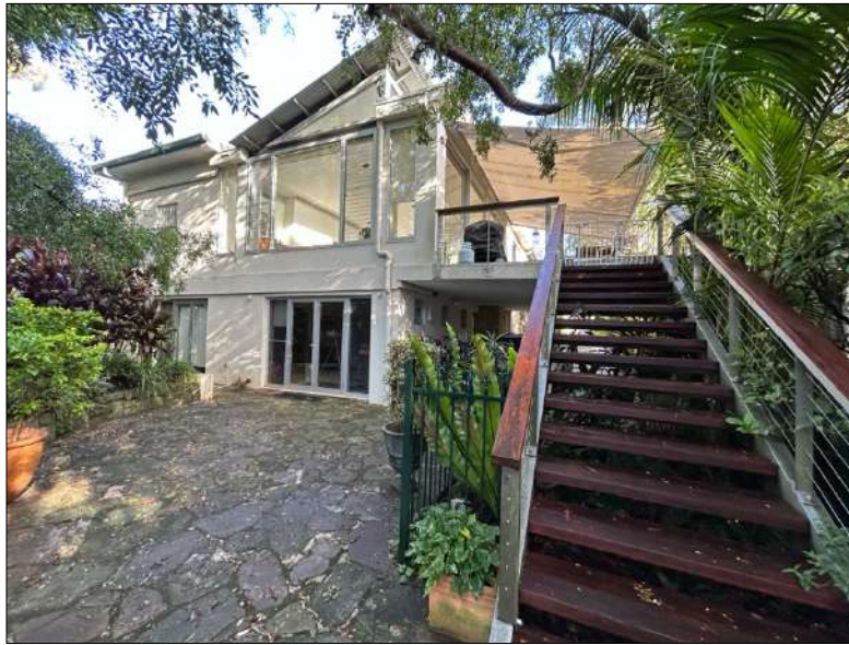
Figure 34: Rear of the dwelling. Clayton Woods of ESEA.
