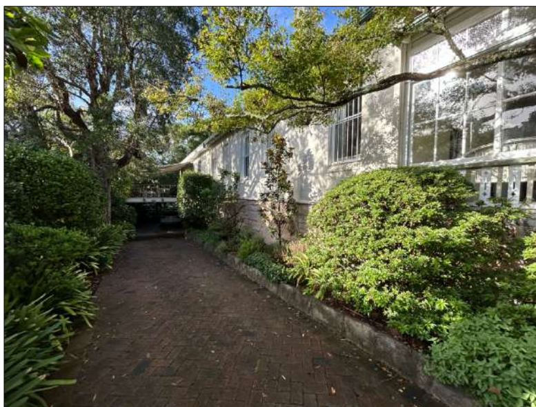
Figure 33: North eastern elevation of the dwelling and the driveway. Clayton Woods of ESEA.
